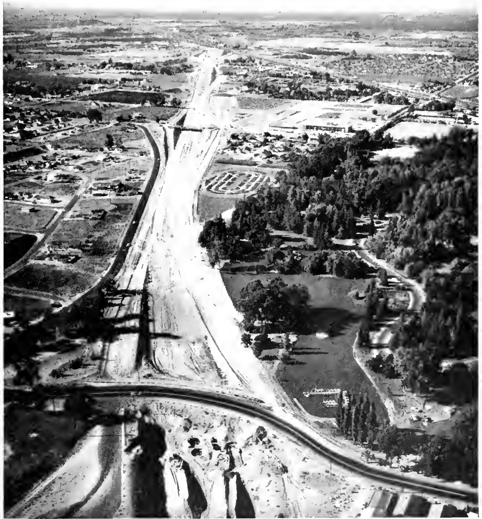
Looking north on Fresno Freeway, showing construction
